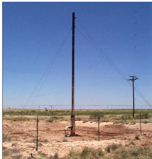
Figure 6. A gas vent and protective pit.
